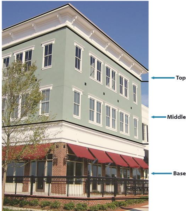
Figure 2.2.11-2: Building Façade Elements
