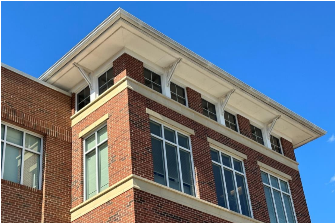
Figure 2.2.11-3: Roof Parapet Wall and Cornice Treatment
