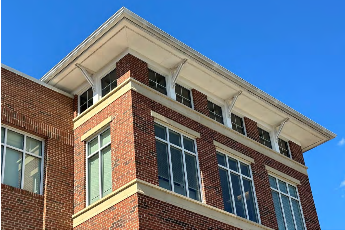
Figure 2.3.6-3: Roof Parapet Wall and Cornice Treatment
