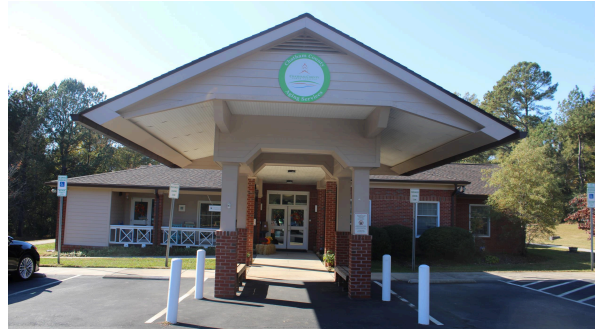
Picture: Pittsboro Center for Active Living
