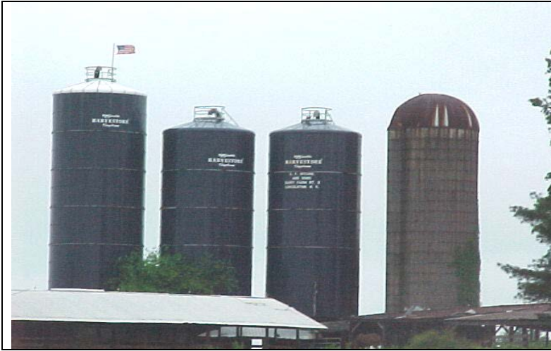
MS 25/59 SILO CON. STAVE AND GLASS LINED
