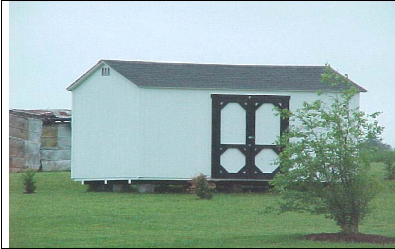
MS 28 STORAGE BUILDING
