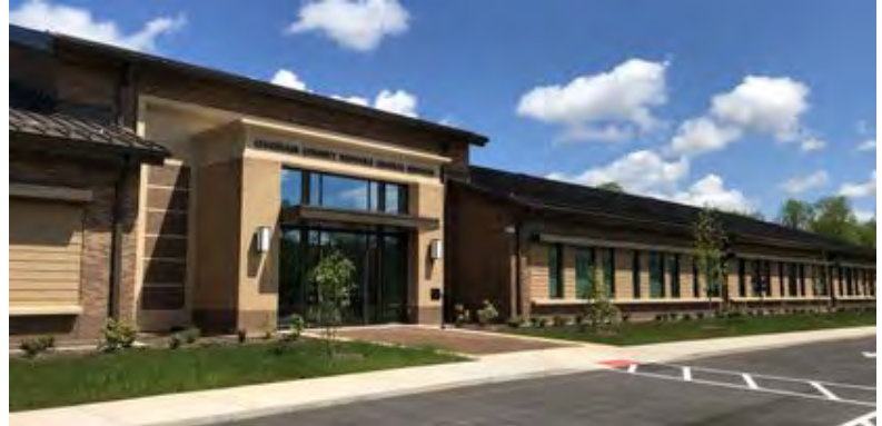
The recently completed Central Services Building for Chatham County Schools located at 468 Renaissance Dr
