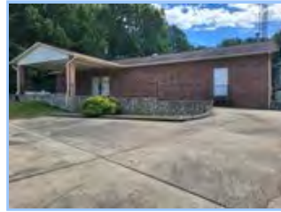
Current Backup EOC
