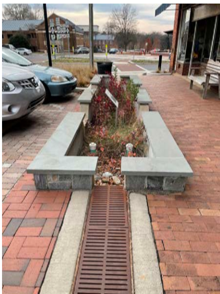
A bioretention cell in downtown Pittsboro that captures and treats stormwater runoff.
