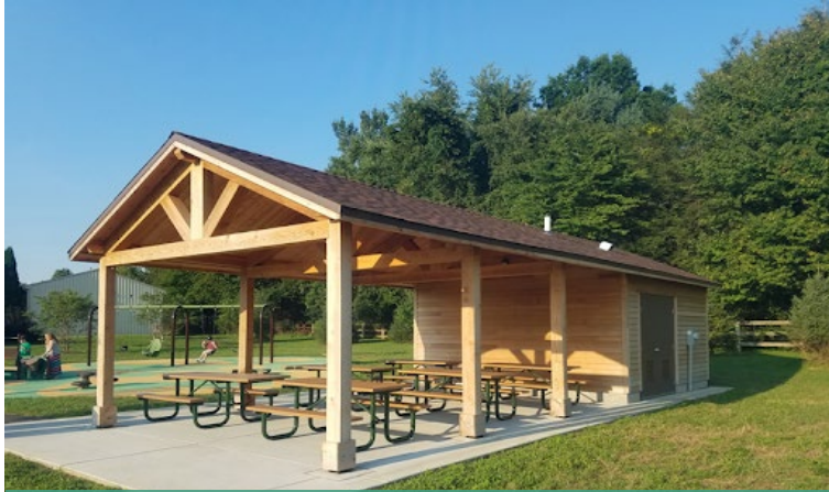
Shelter with restrooms
