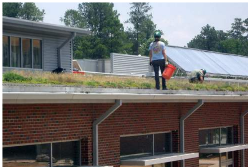
Green Roof on central carolina community college's Sustainable technologies center
