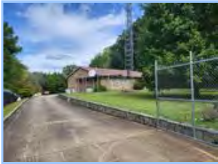
Current Backup EOC
