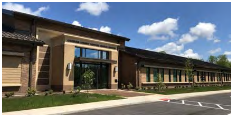
The recently completed Central Services Building for Chatham County Schools located at 468 Renaissance Dr
