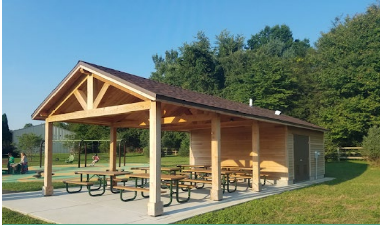
Shelter with restrooms
