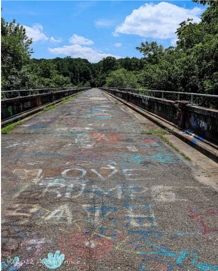
Old Bynum Bridge
