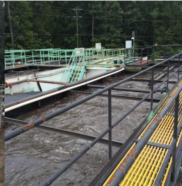
Governors Club 300,000gpd WWTF designed exclusively for Governors Club development, K-8 School, & potential North Chatham High School
