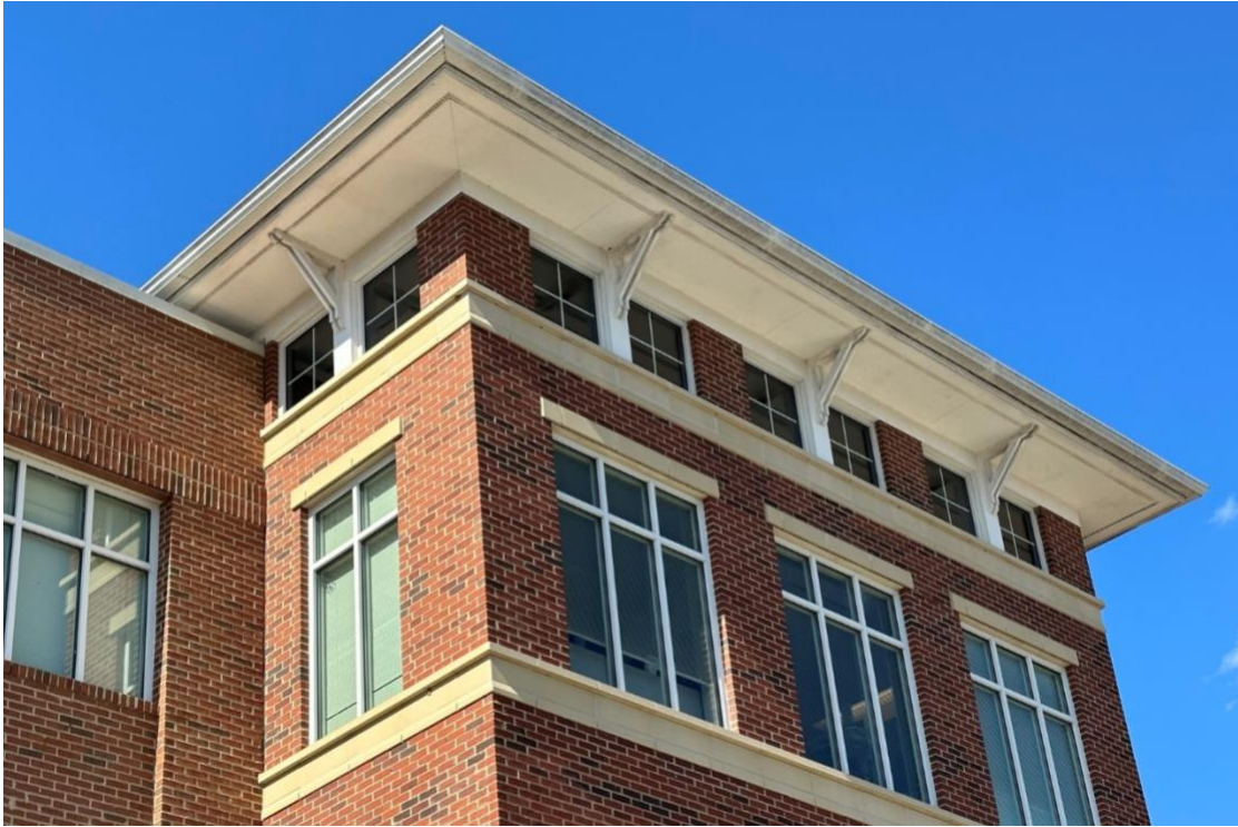
Figure 2.2.11-3: Roof Parapet Wall and Cornice Treatment
