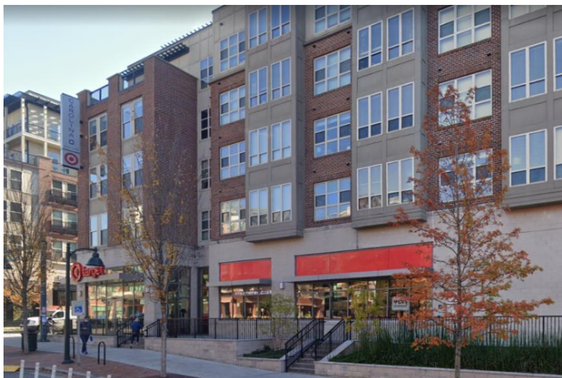
Figure 2.2.11-1: Front Façade Offsets
