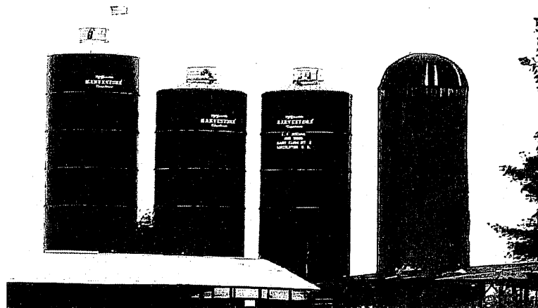
MS 25/59 SILO CON. STAVE AND GLASS LINED
