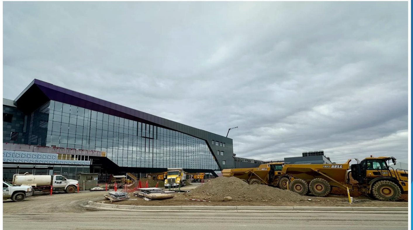
Wolfspeed's under-construction factory in Siler City, N.C. Photo: Zachery Eanes/Axios
