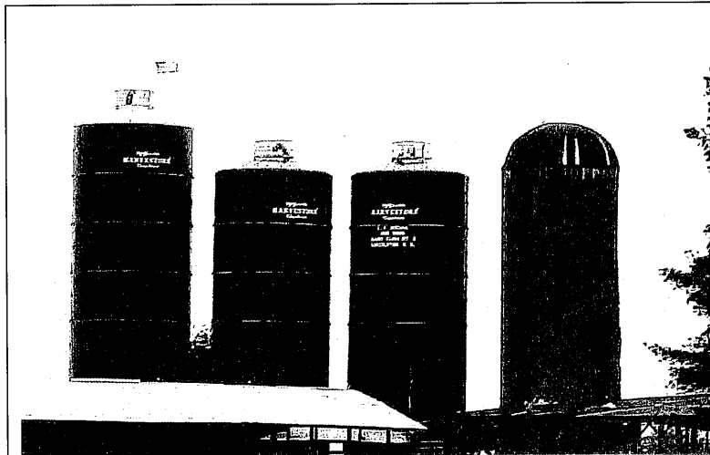
MS 25/59 SILO CON. STAVE AND GLASS LINED
